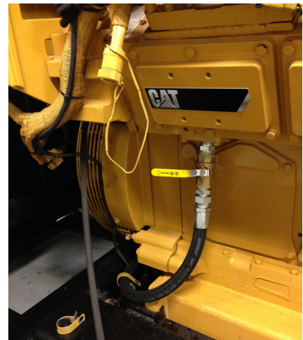
Figure 5. The test engine's left side showing CSM supply port. The supply port is mounted to the opposite side to ensure even heat distribution.
