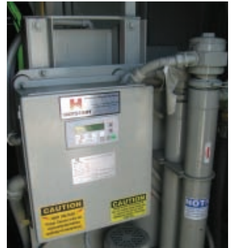
The Kim Hotstart System allows the engine to be plugged into the power grid for easy start-up.
